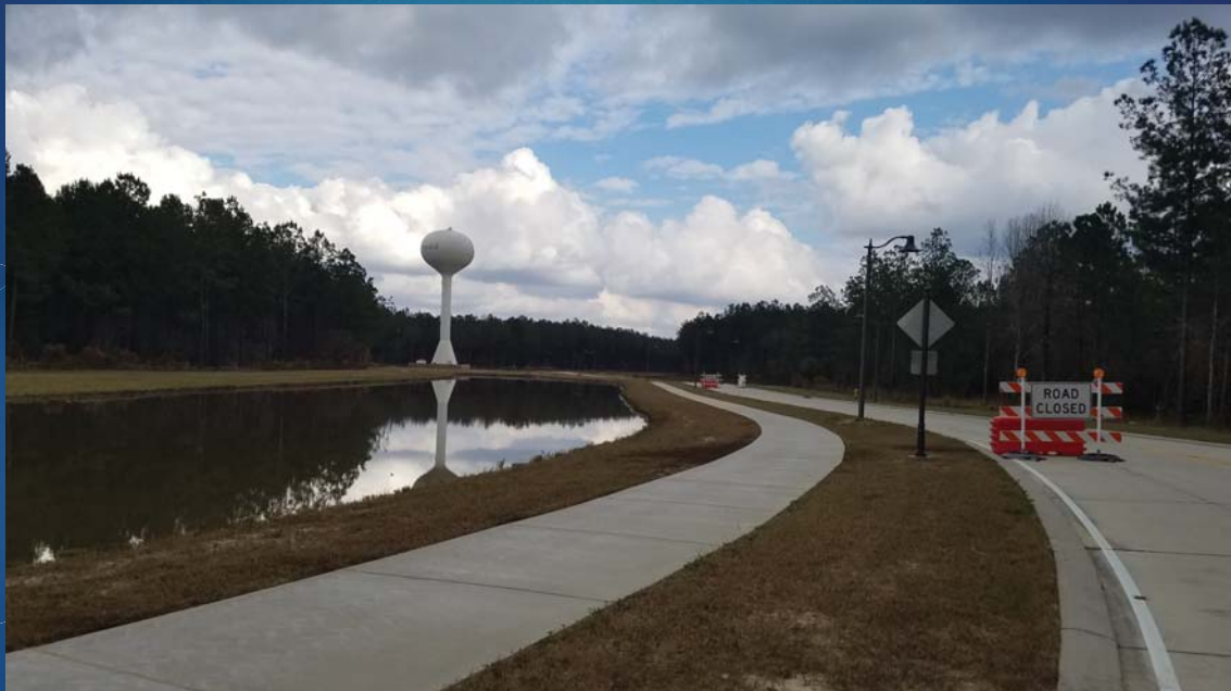
New Water tower at Tamenend development
