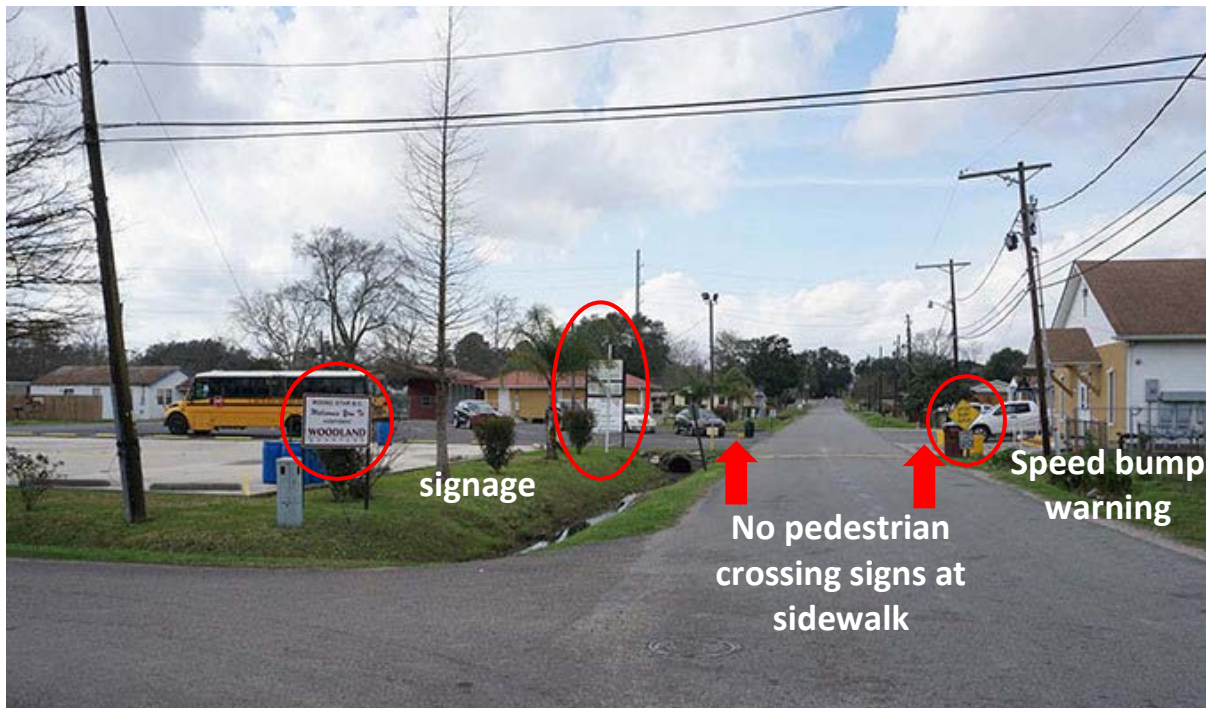
Image 13 – Cardinal St./Dove St. – inconsistent signage, open drainage, overhead utilities, missing crosswalks Photo Credit: DDG 2/14/17
