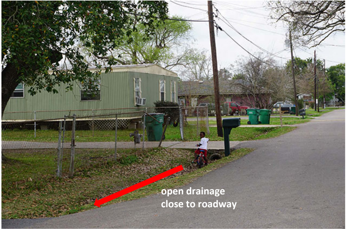
Image 39 – Dove St. - open drainage, overhead utilities Photo Credit: DDG 2/14/17
