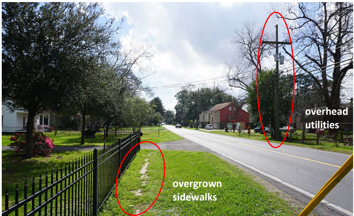
Image 33 – E. 5 th St. – overgrown and damaged sidewalks, overhead utilities, and driveway conflicts Photo Credit: DDG 2/14/17
