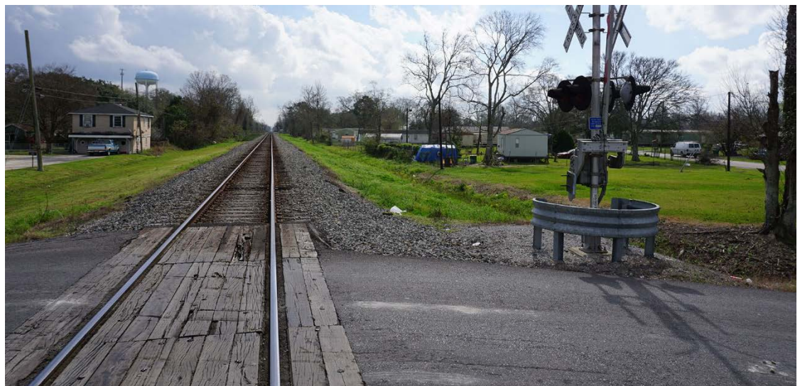
Image 6 – Cardinal Street Railroad Crossing
