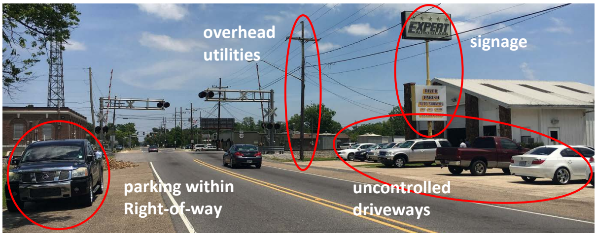
Image 32 – Main St. - overhead utilities, driveway conflicts, uncontrolled parking Photo Credit: DDG 2/14/17
