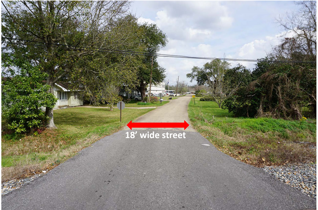
Image 22 – Robin St. - overhead utilities, narrow right-of-way, narrow street Photo Credit: DDG 2/14/17
