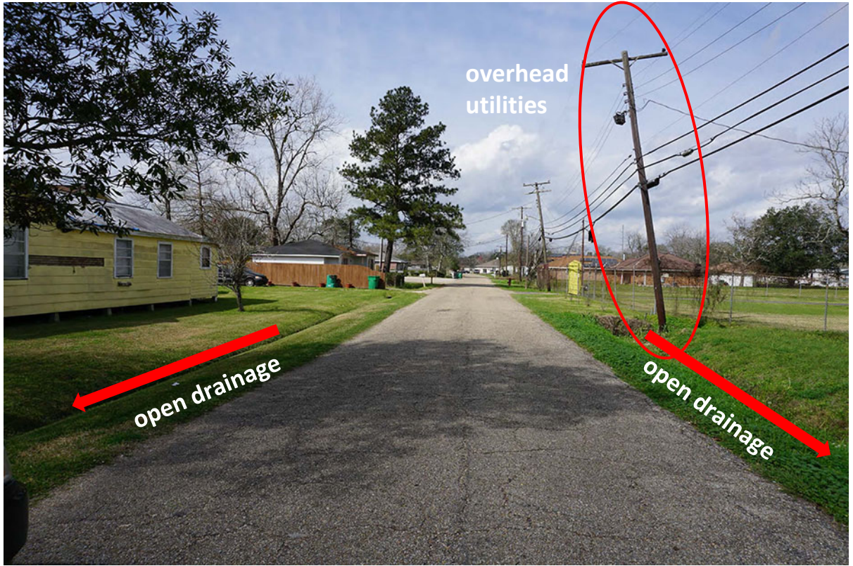
Image 26 – W. 3 rd Street - overhead utilities, open drainage, large right-of-way Photo Credit: DDG 2/14/17
