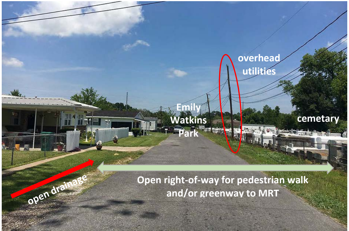
Image 20 – Redbud St. - overhead utilities, larger right-of-way, and few conflicts Photo Credit: DDG 5/10/17
