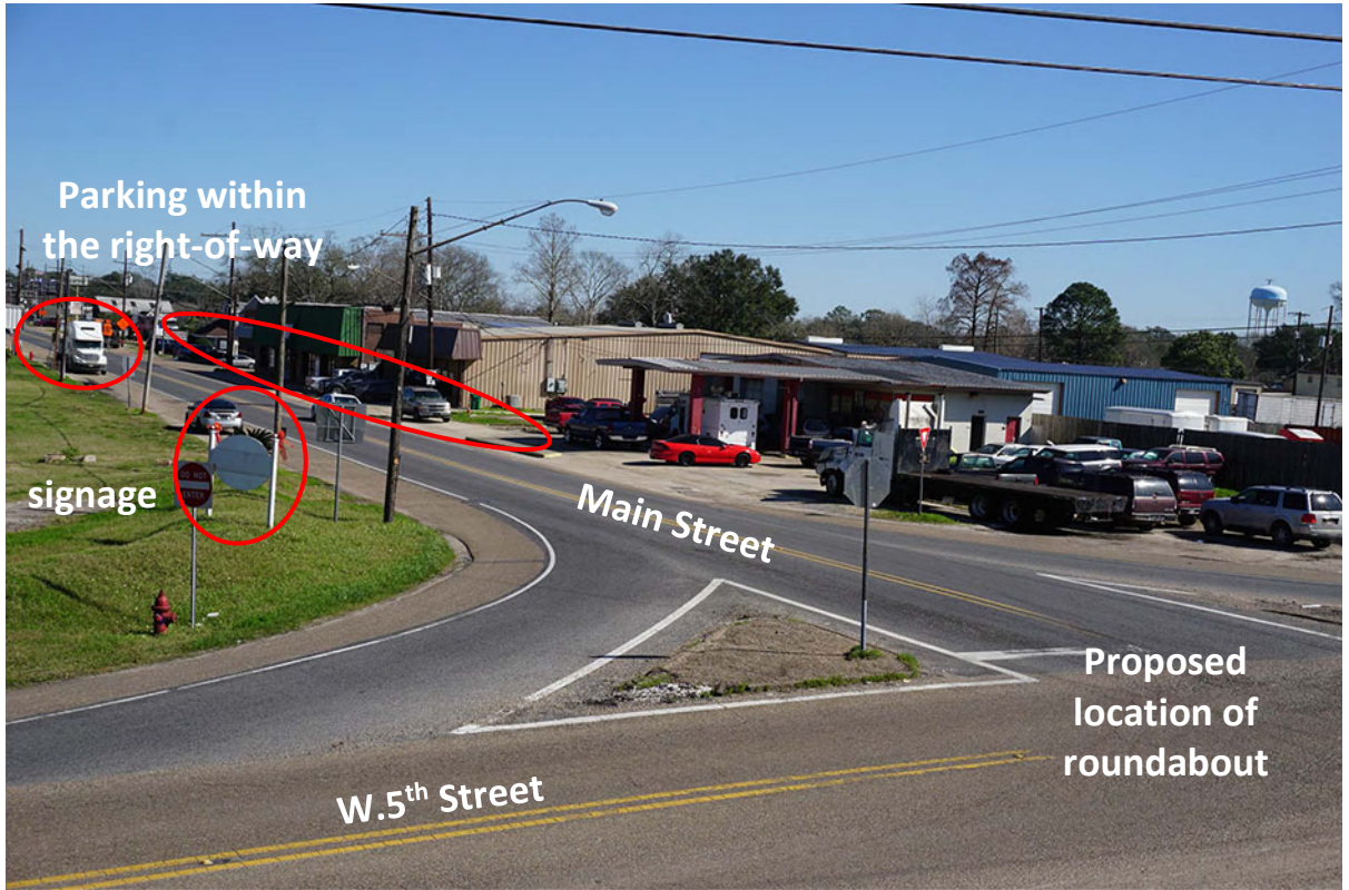
Image 16 – Main Street/5 th Street - overhead utilities, uncontrolled parking, and inconsistent signage Photo Credit: DDG 2/14/17
