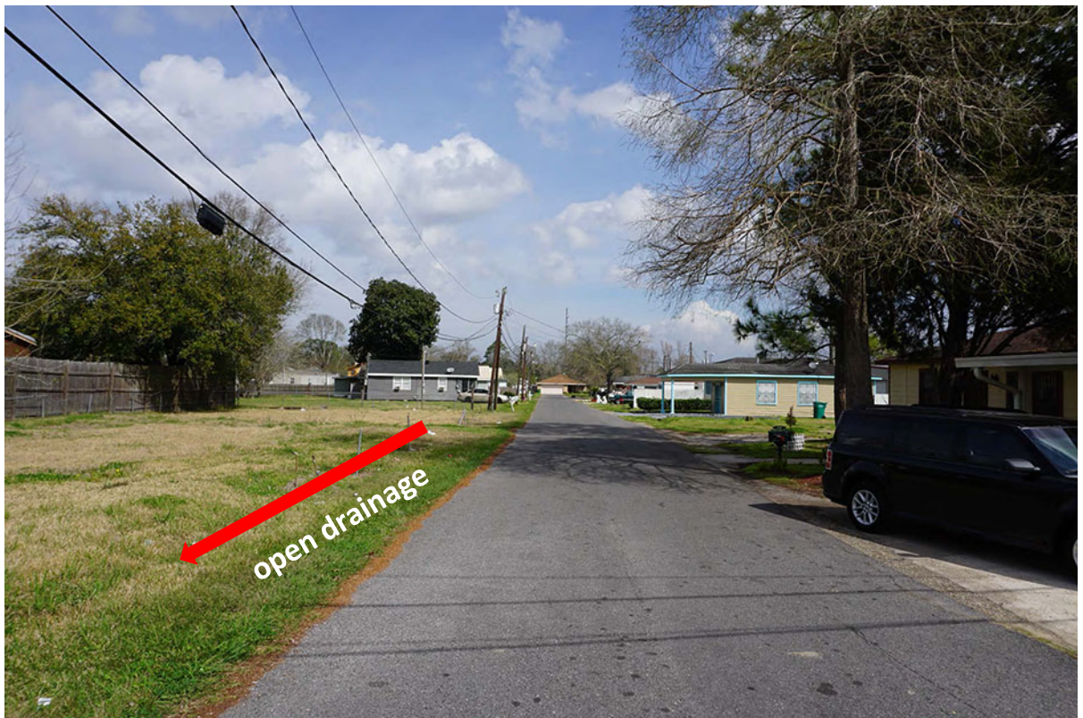
Image 23 – Satsuma St. - overhead utilities, narrow right-of-way, and visibility issues at 2 nd street Photo Credit: DDG 2/14/17
