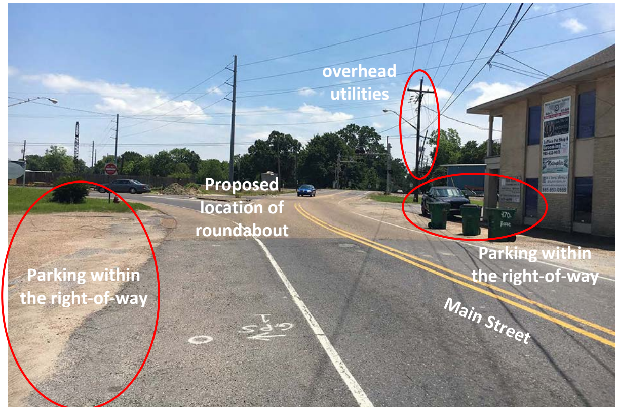
Image 15 – Main Street/5 th Street - overhead utilities, uncontrolled parking, and inconsistent signage Photo Credit: DDG 2/14/17
