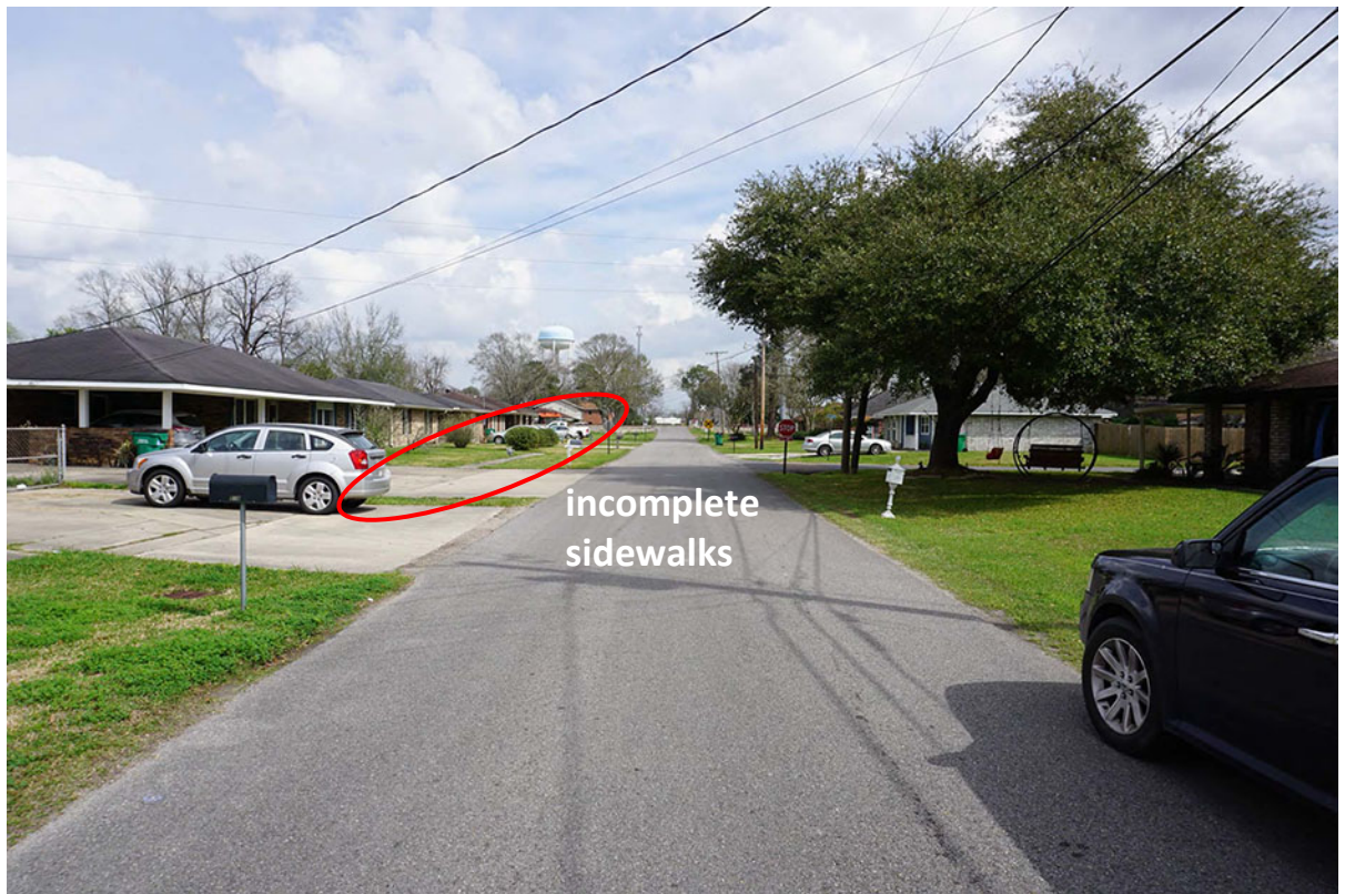
Image 31 – Walnut St. - overhead utilities, subsurface drainage, driveway conflicts, incomplete sidewalks Photo Credit: DDG 2/14/17
