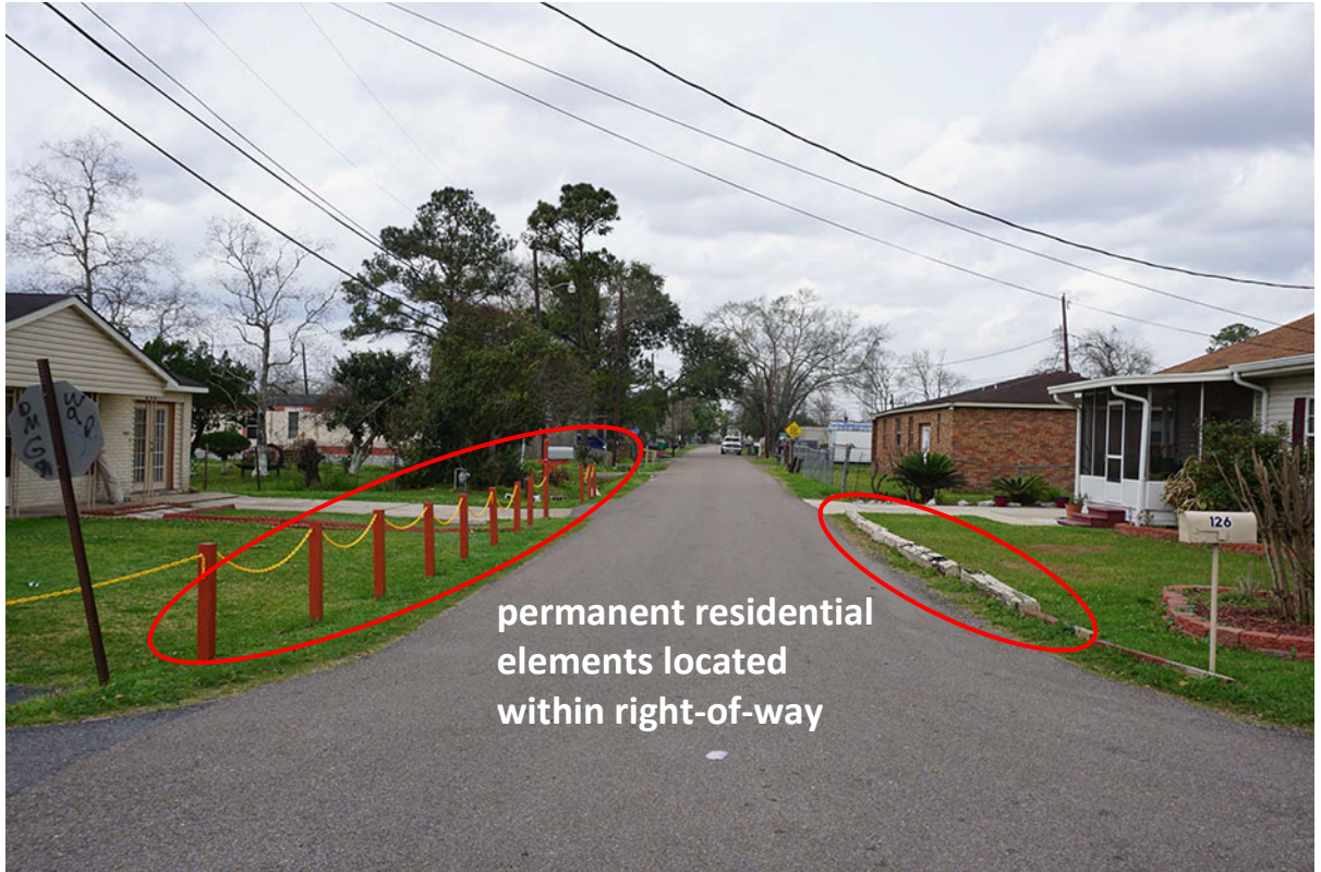
Image 24 – Dove St. - overhead utilities, encroachment within the right-of-way created by residents Photo Credit: DDG 2/14/17
