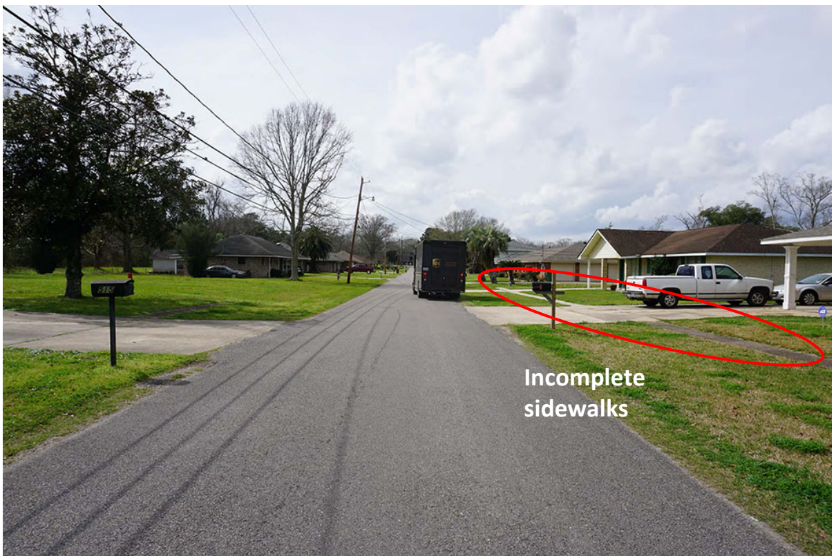
Image 35 – Walnut St. – incomplete sidewalks, overhead utilities, and driveway conflicts Photo Credit: DDG 2/14/17
