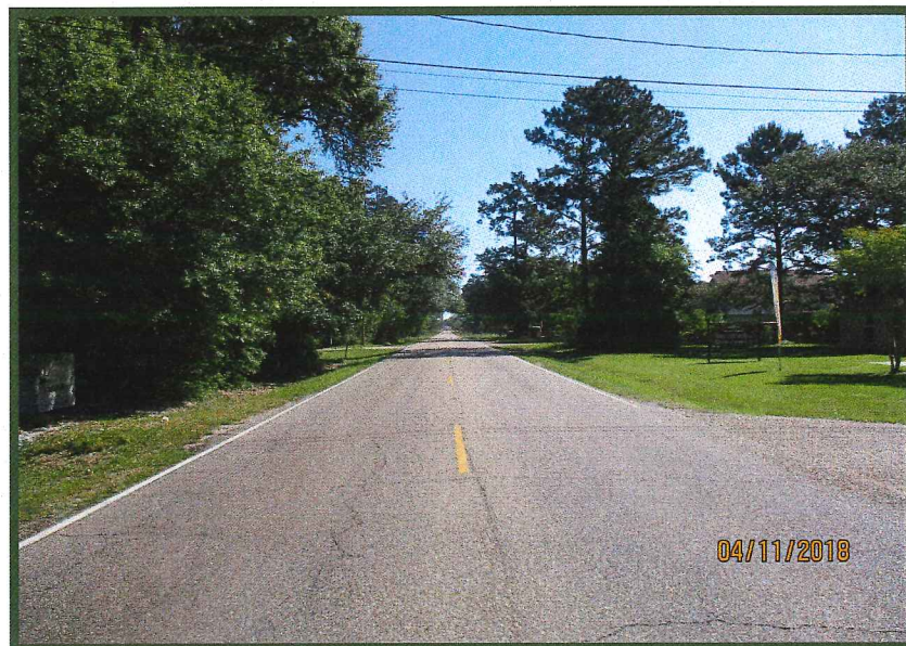
Figure 1.2 – LA 1040 – Existing Conditions – Klein Drive to Old Baton Rouge Highway
