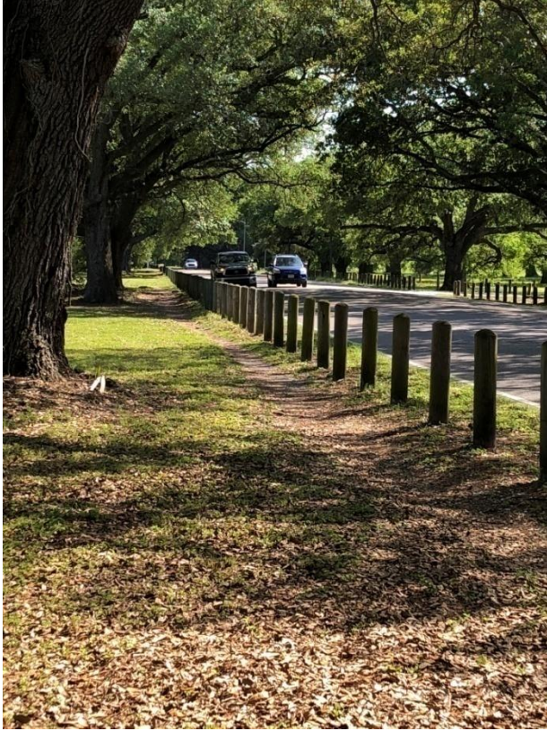
Photo 9: Lack of sidewalk along Marconi Drive has led to pedestrians wearing a path.
