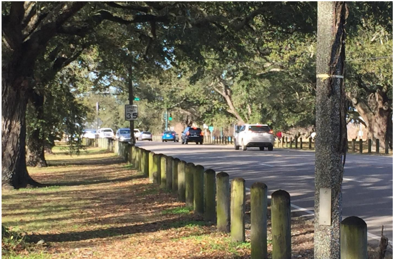
Photo 5: Wood bollards at edge of road to deter parking under trees.
