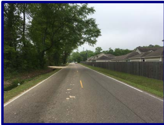
Figure 6.6 - Existing Street View along Minnesota Park Road Looking West (Source: RCLC)
