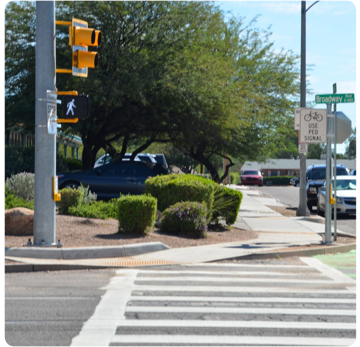
Figure 34 - Crossing Marking with On-Demand Signal
