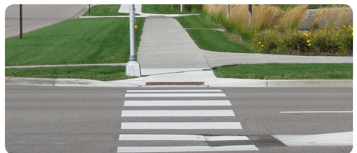
Figure 9 - High-Visibility Crosswalk
