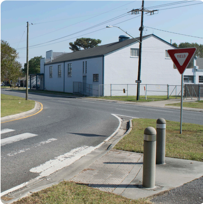
Figure 29 - Vehicular Barrier
