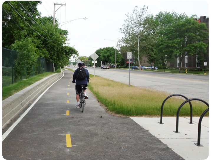
Figure 26 - Shared-Use Trail, Roadway Right-of-Way
