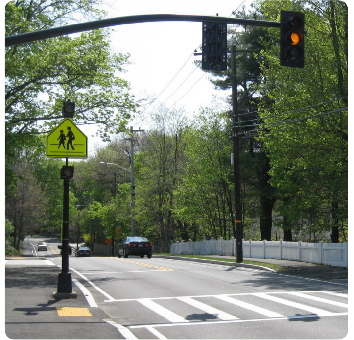
Figure 32 - Active Warning Beacon
