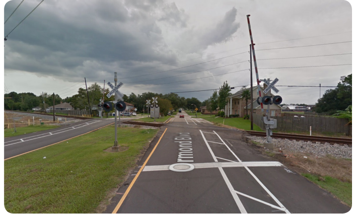
Figure 15- Ormond Boulevard Crossing on the East Bank, facing River Road
