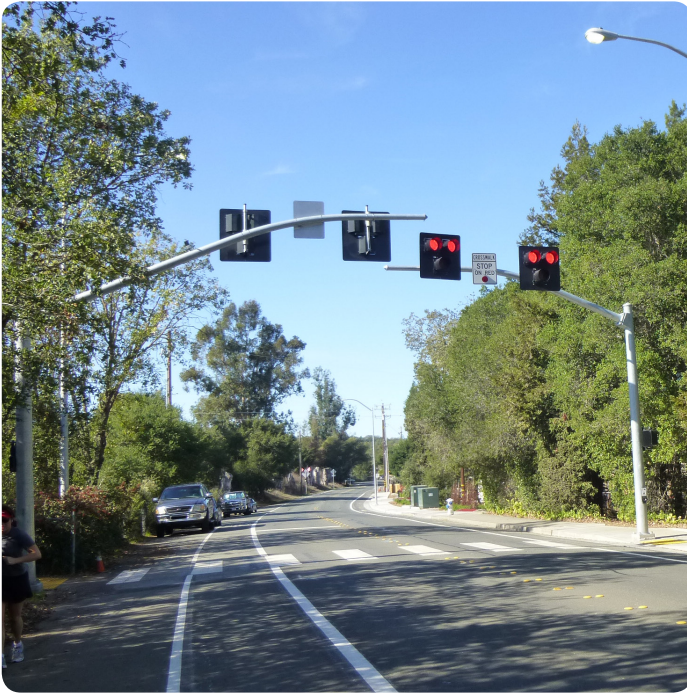
Figure 33 - Hybrid Beacon at Crossing
