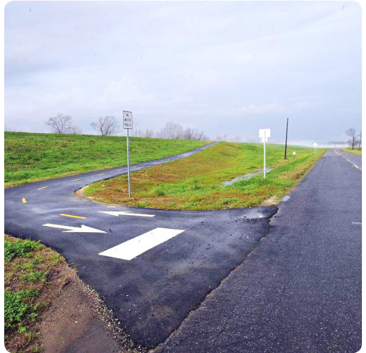
Figure 30 - Levee Access Path
