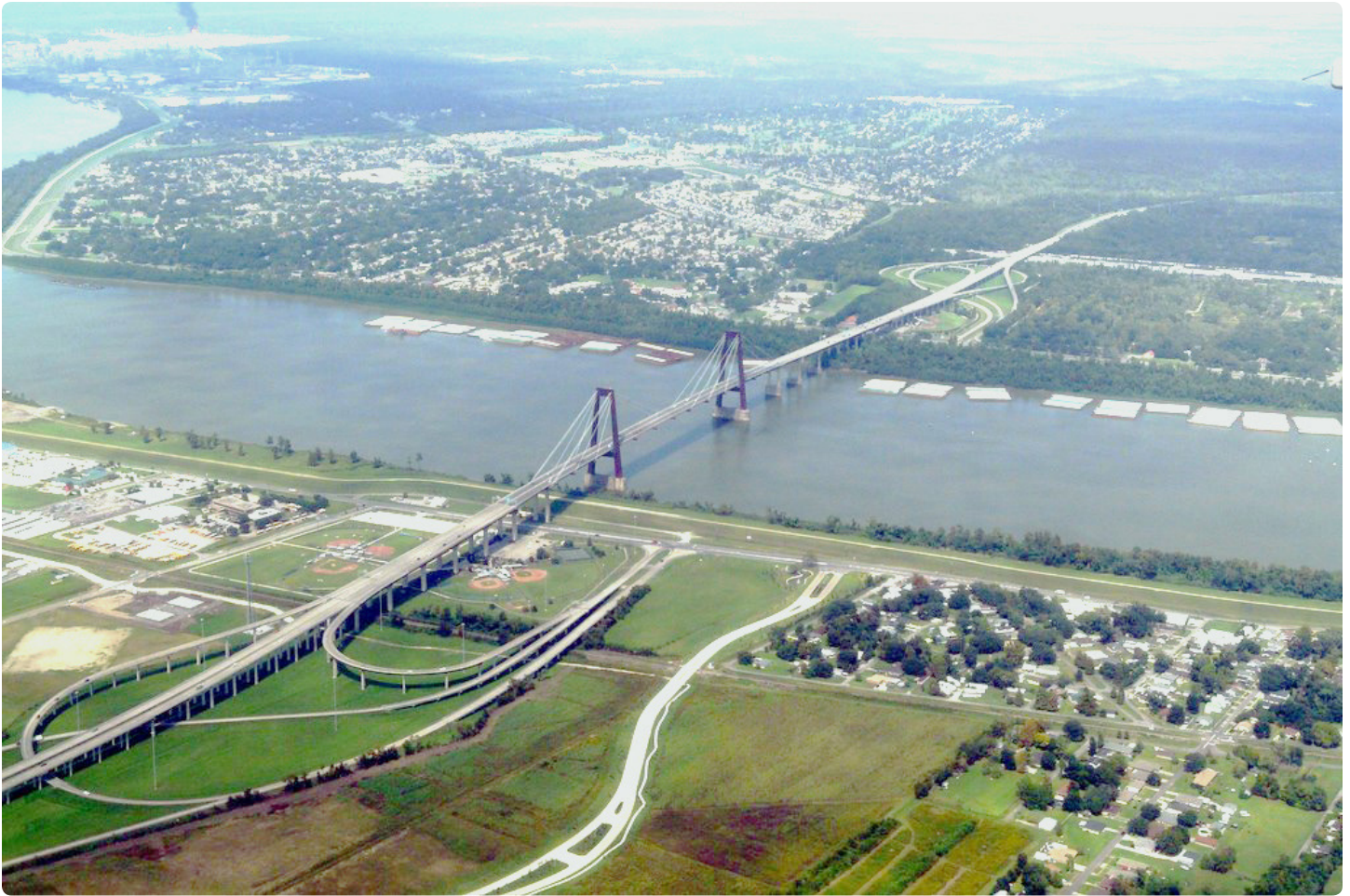
Figure 54 - Aerial View of Hale Boggs Memorial Bridge
