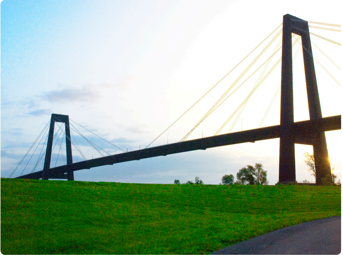
Figure 2 - Hale Boggs Memorial Bridge in Luling
