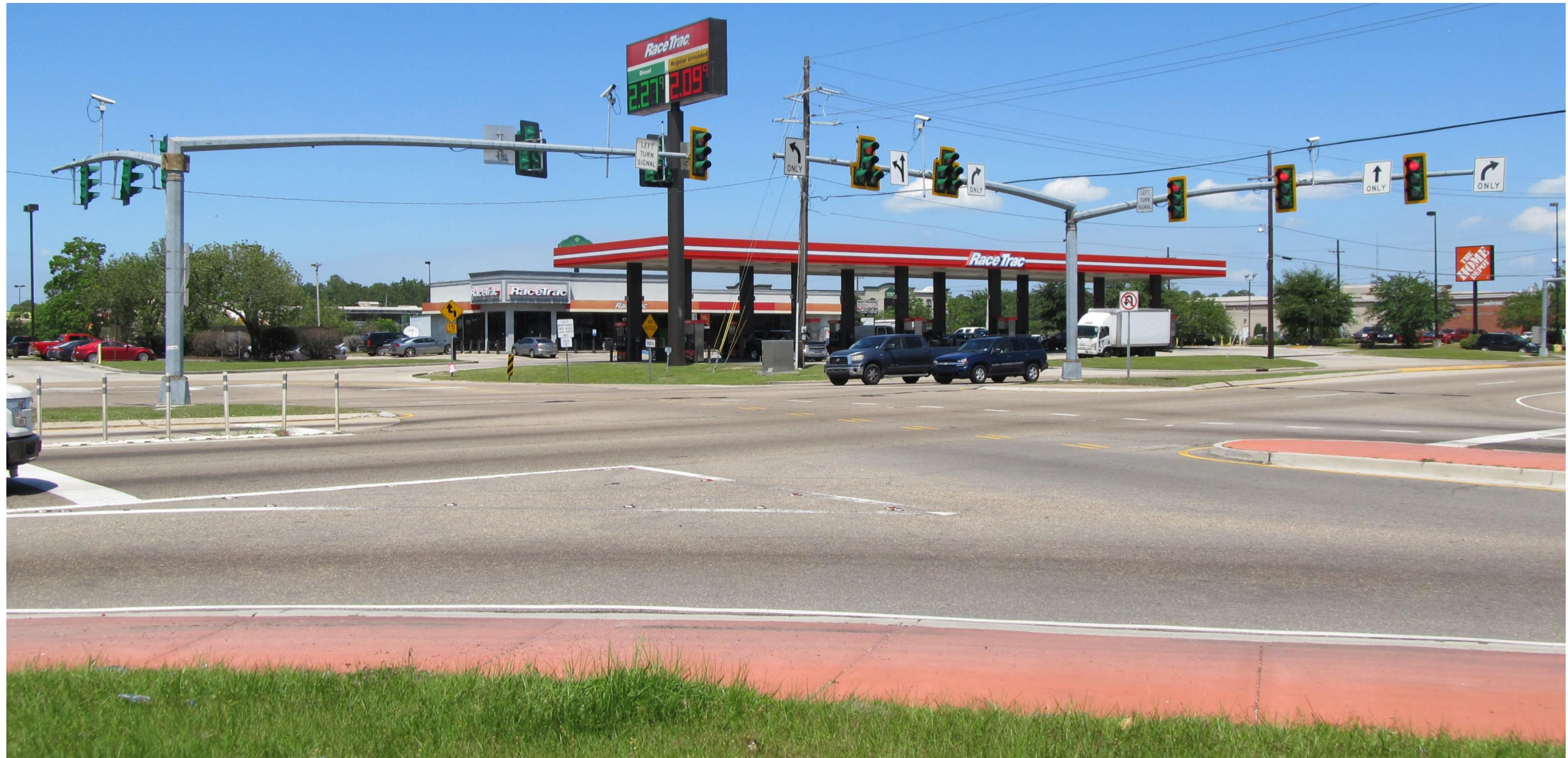
FIGURE 7 – US 190 (GAUSE BOULEVARD) @ I-10 EAST SERVICE ROAD/TYLER STREET
