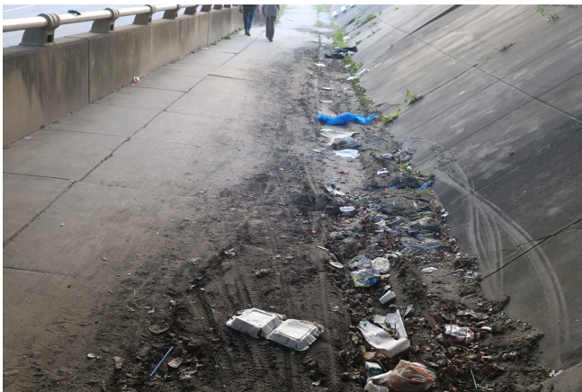
Dirt, silt, debris, and litter collect at the base of concrete retaining walls, covering significant portions of the underpass sidewalk.
