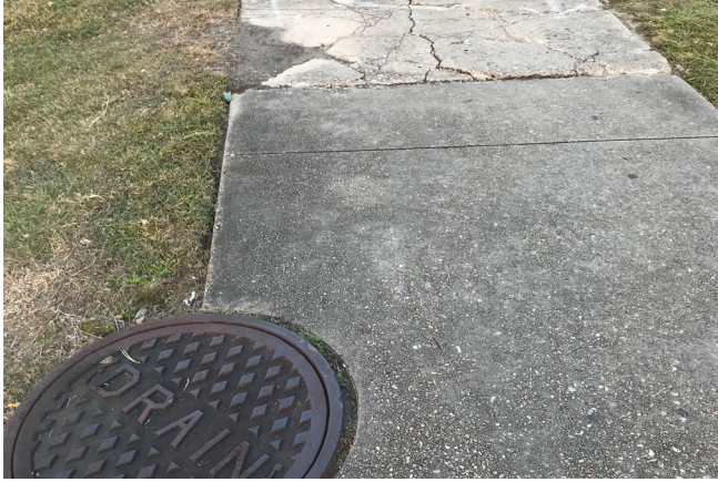
A drainage system access point encroaches onto the sidewalk.
