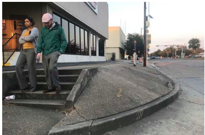
The sidewalk on the upriver side of the avenue is interrupted by a short set of stairs that are not accessible to people in wheeled mobility devices.
