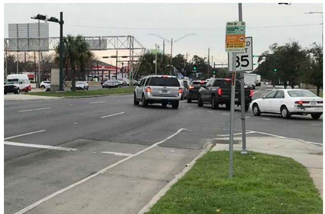
Signed bus stop at South Carrollton Avenue and Dixon Street does not provide any concrete access pad to the sidewalk for people using mobility assistance devices.
