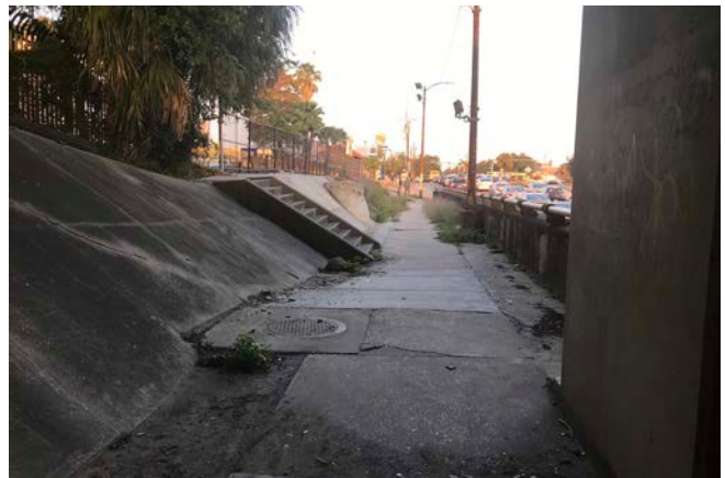
The retaining walls for the expressway, railroad bridge, and adjacent parcels are covered in concrete and include remnant staircases that presumably provided access to now fenced off parcels or a prior pedestrian route.
