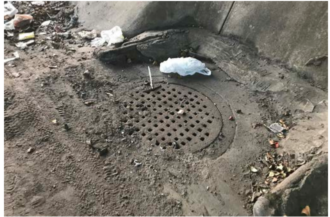
A drainage area under the express shows where dirt, silt, and debris collect along the base of a retaining wall on the north side of South Carrollton Avenue.
