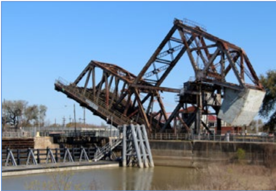
Historic St. Claude Bridge, a 1919 Strauss heel trunnion bascule bridge in operation over the IHNC lock Photo: LA DOTD Louisiana Historic Bridge Inventory
