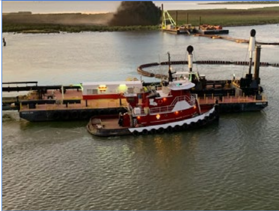
Dredging operation with flume of sand as beneficial use /land creation near SW Pass
