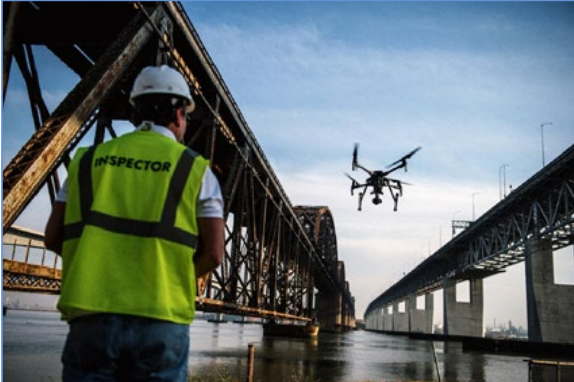
Railroads and highway departments are beginning to use drones to conduct bridge inspections Photo: dan_hennage_lr
