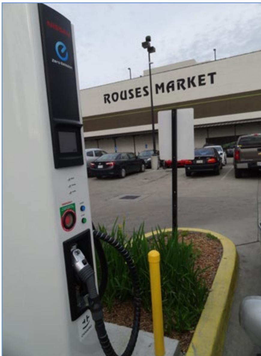
Direct current or DC fast charger for battery electric vehicles (EV) at local Rouses market
