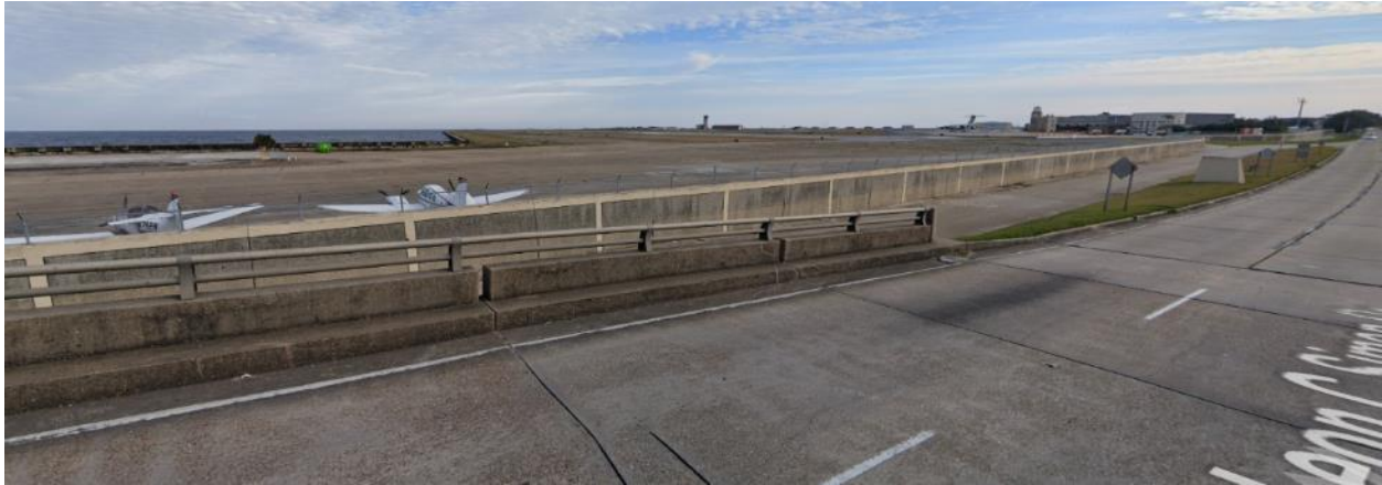
Seabrook Bridge – East of IHNC Near Lakefront Airport
