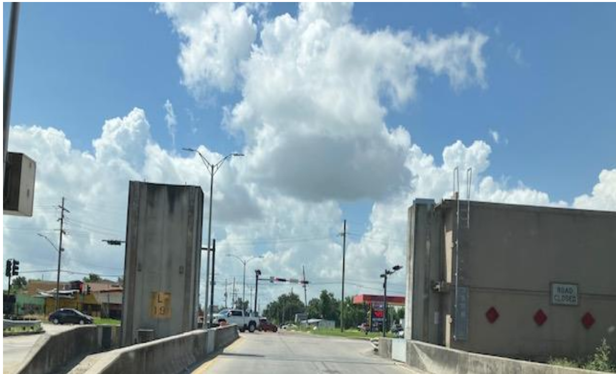
East Access Future Connection – Downman Rd at Railroad Bridge and Floodwall Gate
