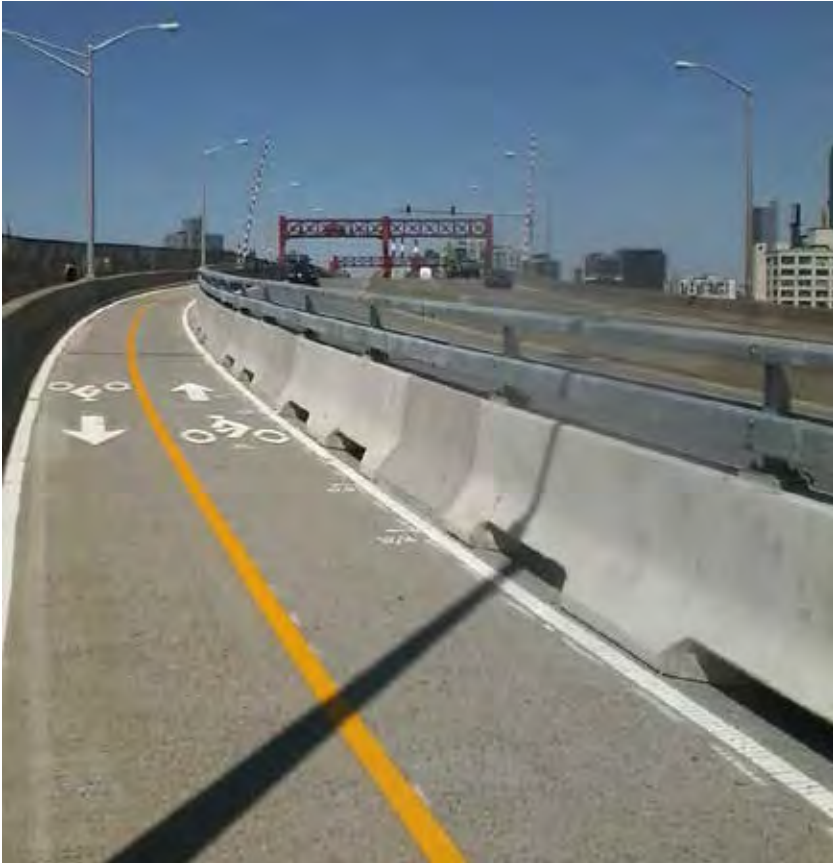
Pulaski Bridge, New York City
