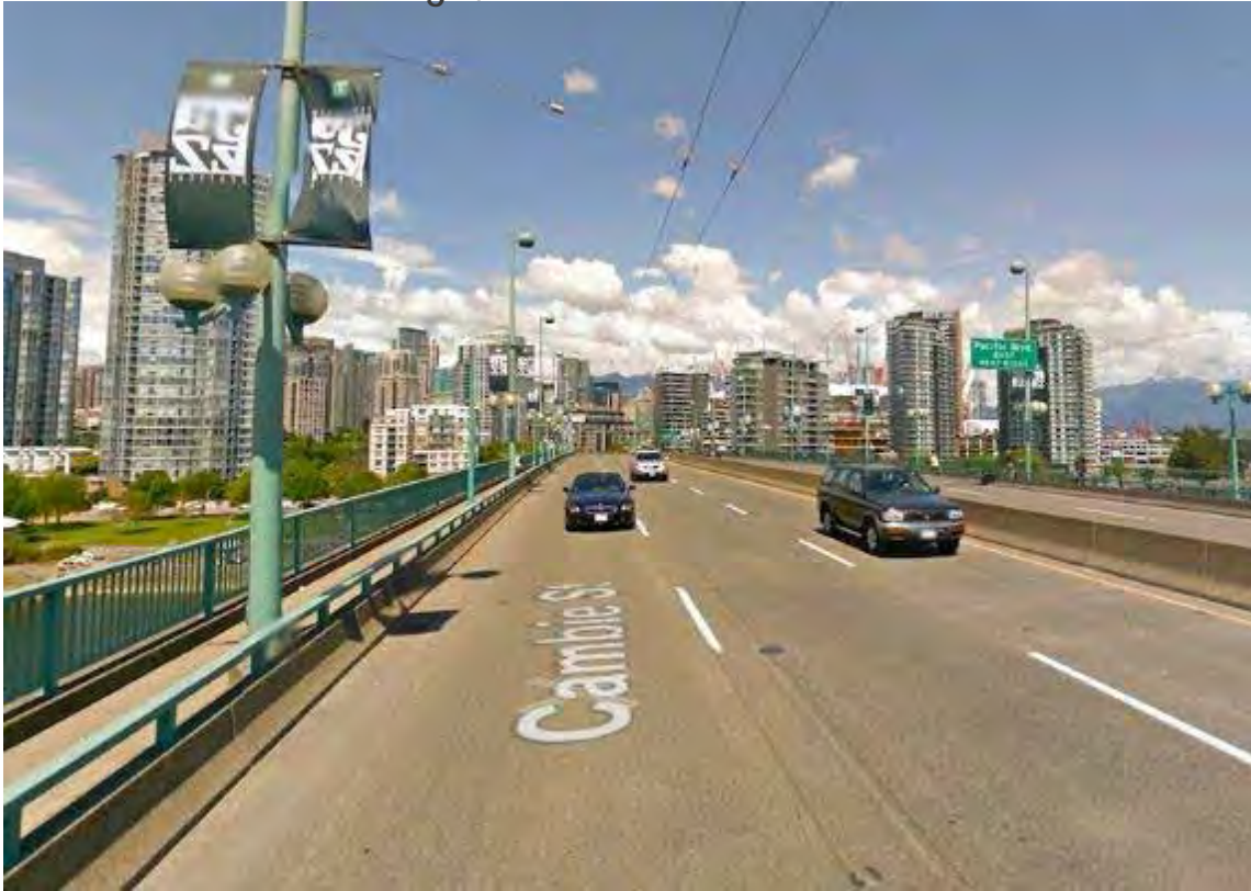
Cambie Street Bridge, before
