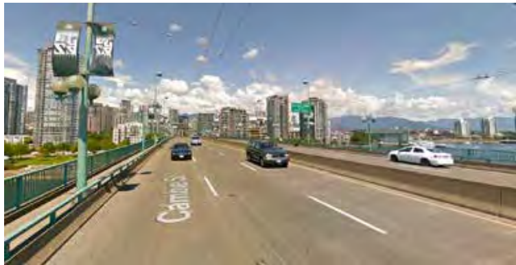
Cambie Street Bridge, before
