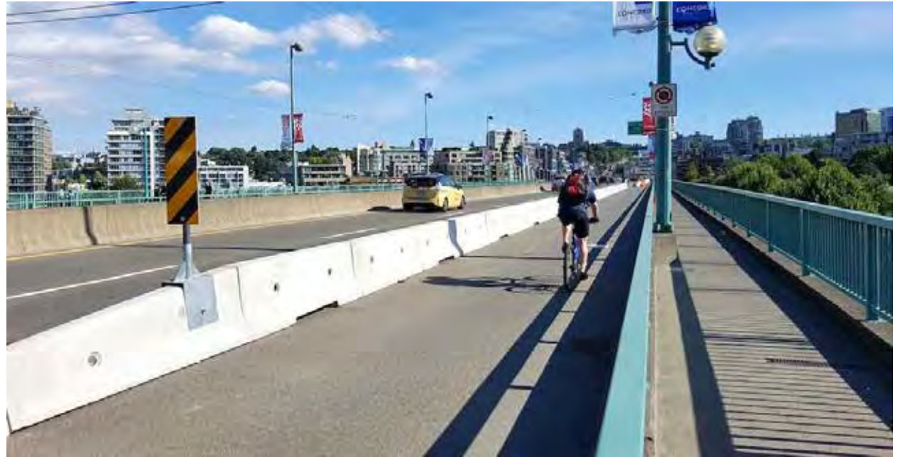
Cambie Street Bridge, Vancouver (after)
