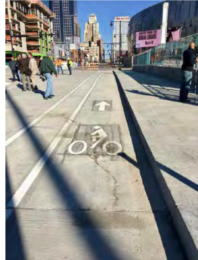
Grand Blvd. Bridge, Kansas City
