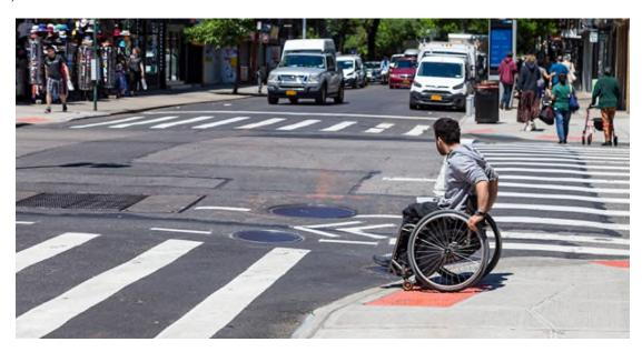
Figure 8-3: ADA Compliant Ramp (Source: nycpedramps)
