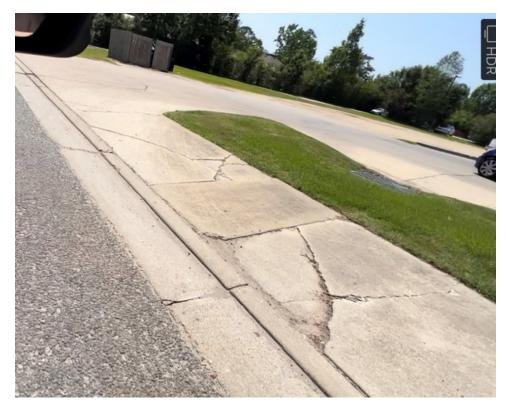
Figure 4-36: Girod Street Cracked Sidewalk Panels
