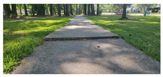
Figure 4-19: Concrete Sidewalk Slab Elevation Differential (Monroe Street)
