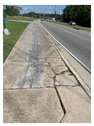
Figure 4-27: Badly Cracked Sidewalk and Elevation Differential (US 190)
