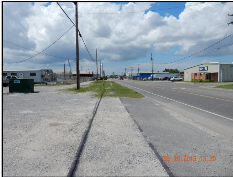
Figure 3-19. View of Hooper Spur Track on Peters Road (view facing south)
