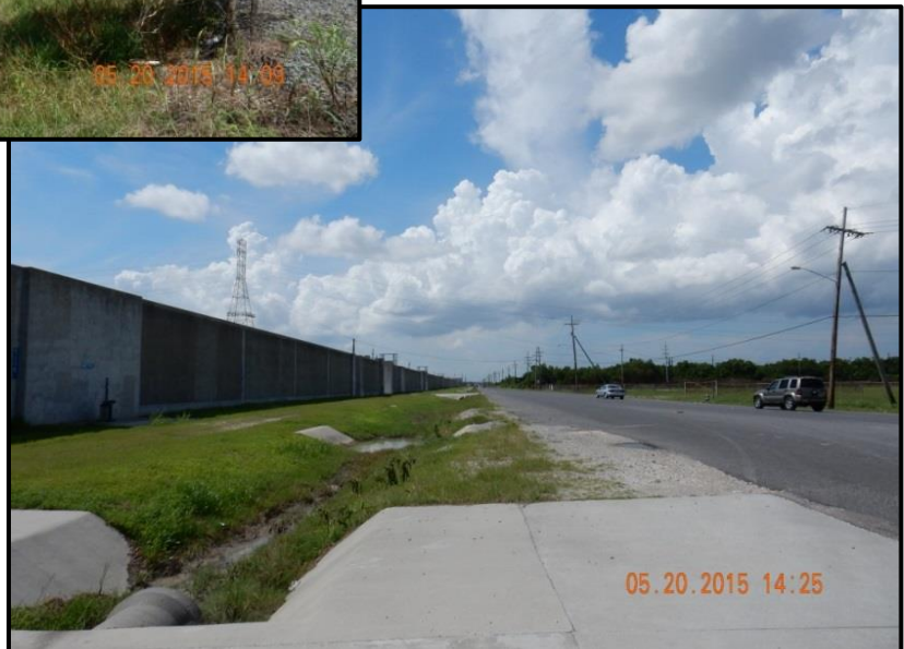
Peters Road south of Lapalco Boulevard adjacent to Boomtown Floodwall (photo right; view facing north)
