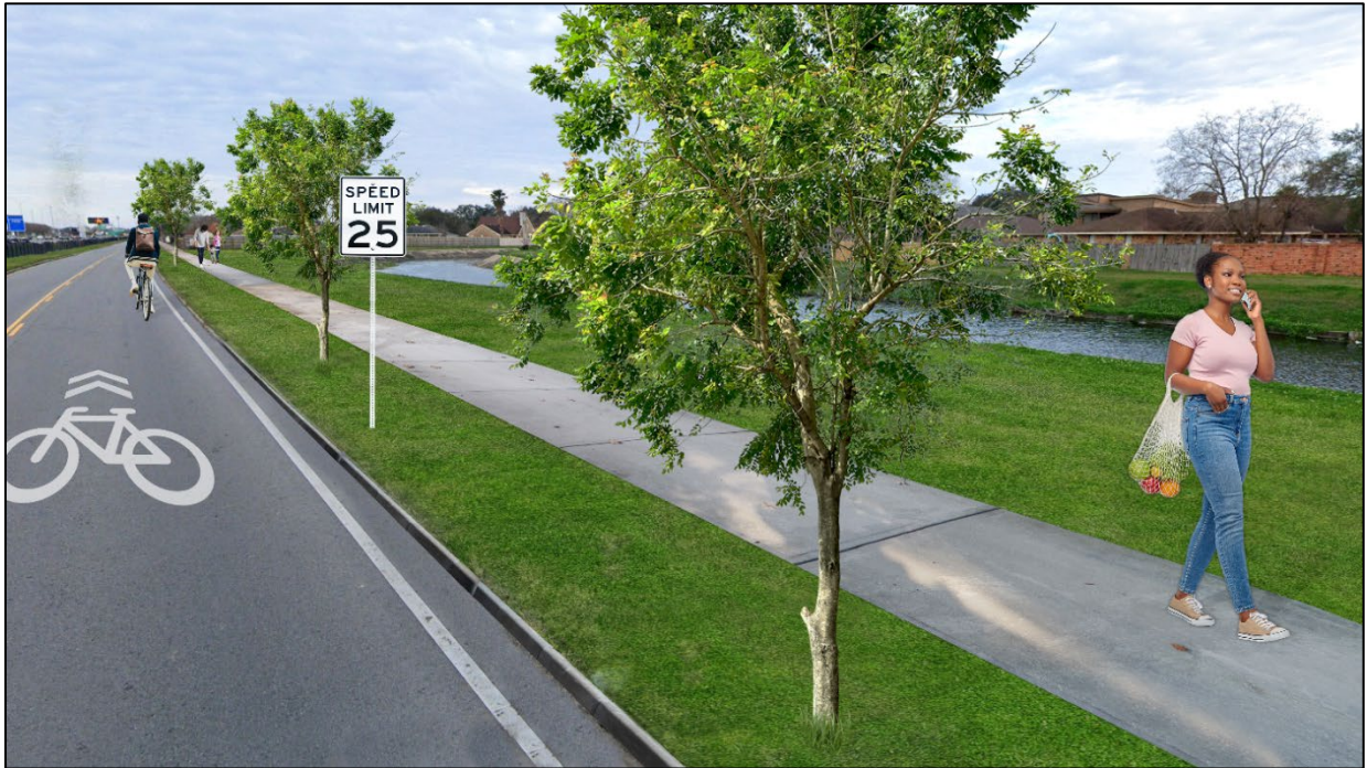
Figure 54: Speed Reduction and Shared Lane on Service Roads with New Off-Road Sidewalk
