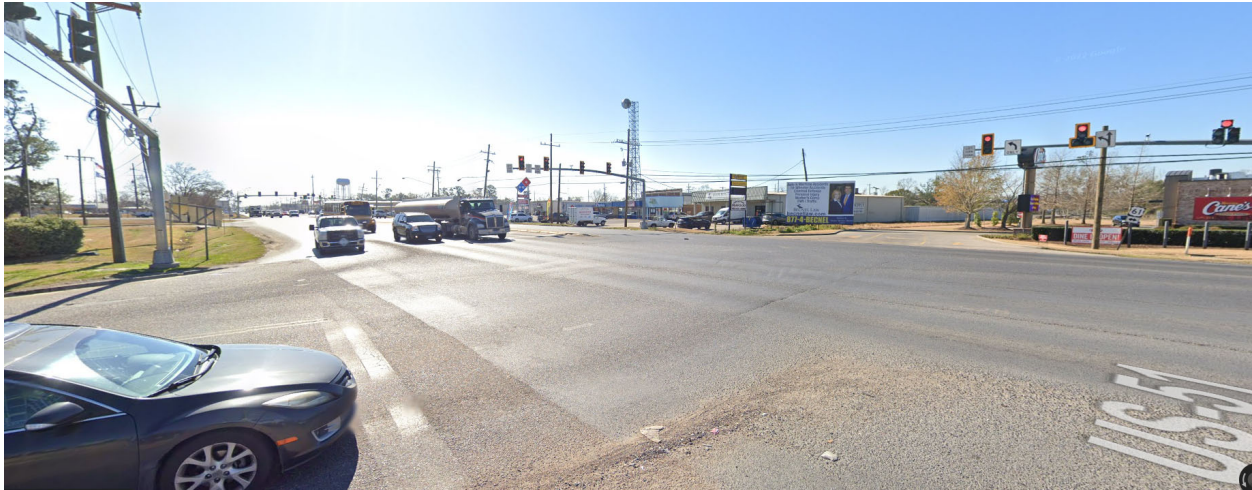
Photo 8 (US 61 at US 51): Lack of crosswalks, pedestrian push buttons, and pedestrian signal heads
