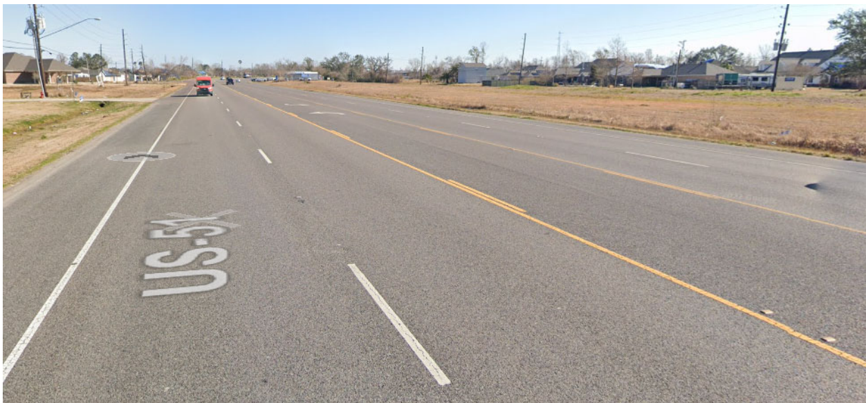
Photo 3 (US 51 between Bamboo Road and Palmetto Drive): Lack of sidewalks, bicycle facilities, and pedestrian refuge along US 51
