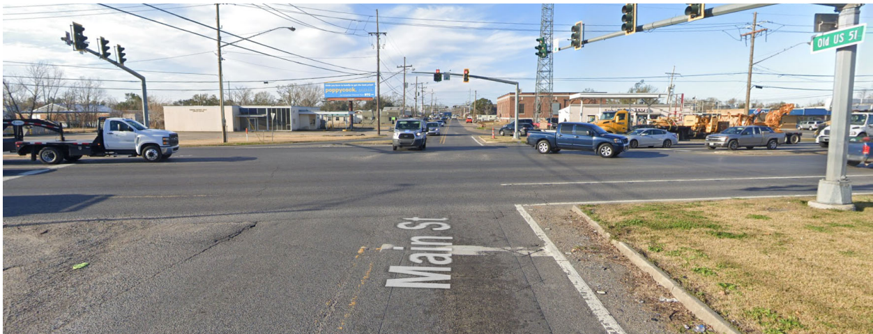
Photo 7 (US 61 at Main Street): Lack of crosswalks, pedestrian push buttons, and pedestrian signal heads
