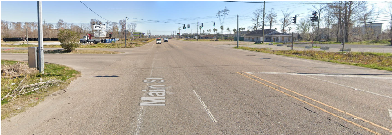
Photo 9 (Woodland Drive at US 51): Lack of crosswalks, pedestrian push buttons, and pedestrian signal heads
