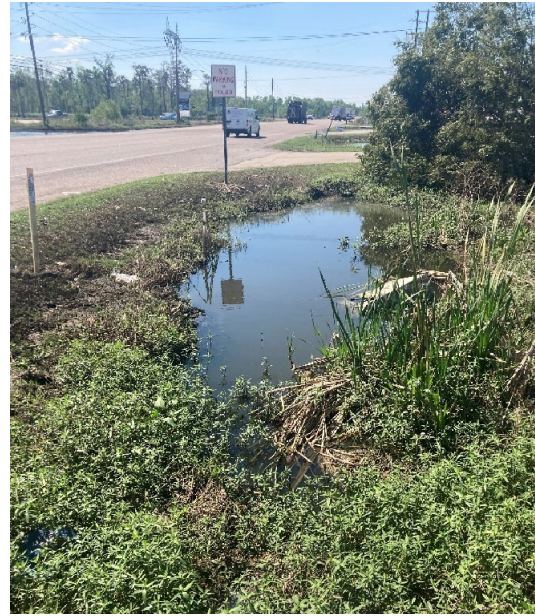
Photo 1: Left - Standing water on the truck entrance to Pilot on Aug 18, 2021, after three days with no rain.
