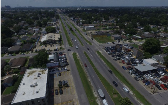
Figure 2: Widening of Causeway Blvd Project
