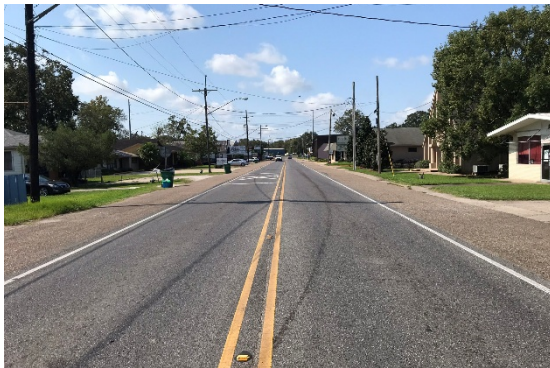
View of Main Street pre-construction
