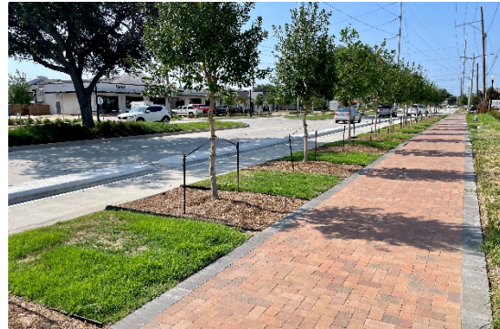
View of Severn Ave. with Improvements
