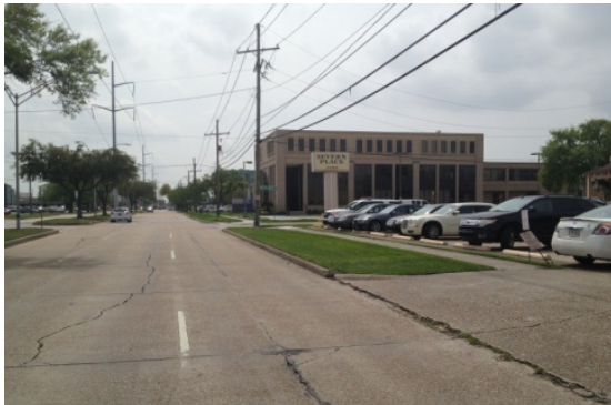
View of Severn Ave. pre-construction
